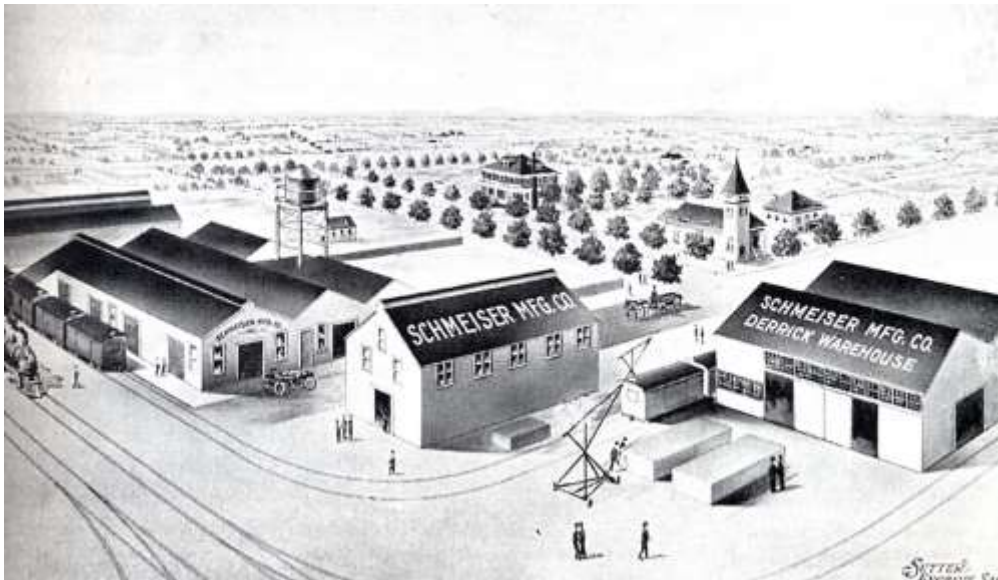
Figure 6: This highly idealized drawing of the Schmeiser Manufacturing Plant, one of Davis' most important non-University related businesses c. 1915. The recently constructed Schmeiser home is seen in the background. The drawing illustrates the close proximity of Old East manufacture and residential.
